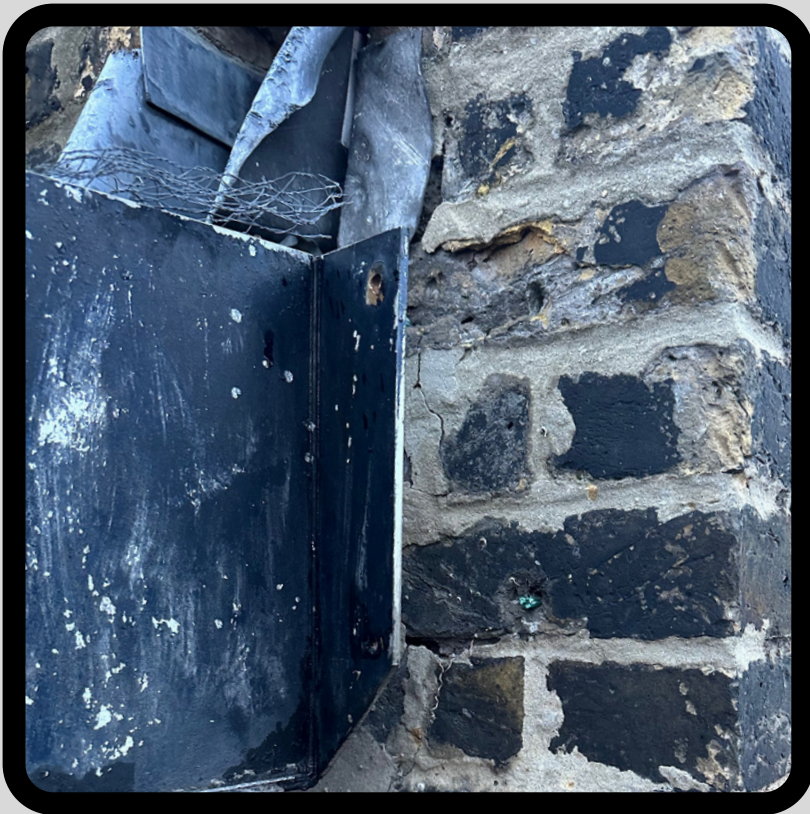
Rear guttering, deterioration and storm damage repair
