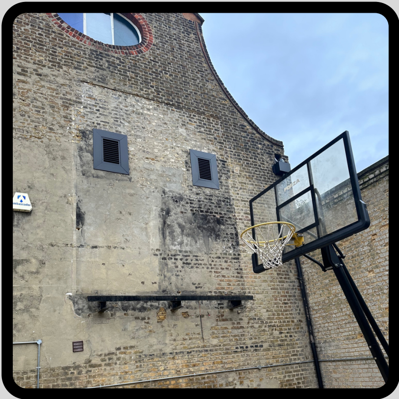
Rear vents for HVAC finished off 2023
